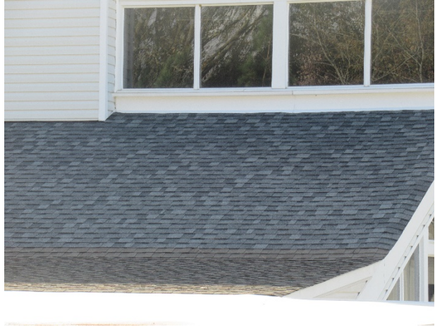
Asphalt shingle roof overview
