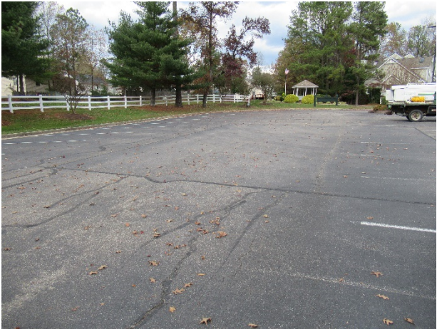
Asphalt pavement overview
