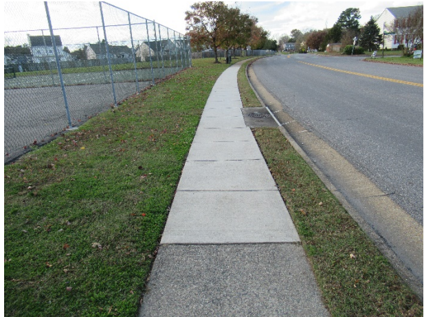
Concrete sidewalk overview
