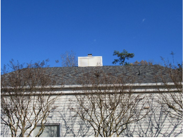
Asphalt shingle roof overview
