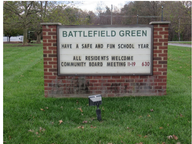
Entrance sign overview – Note: efflorescence
