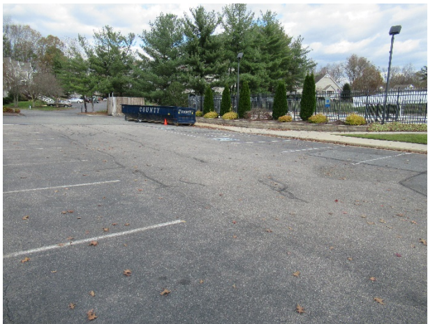
Asphalt pavement overview
