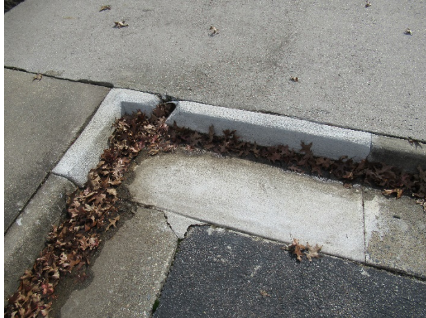
Recently replaced section
