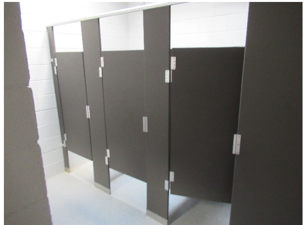
Rest room overview
