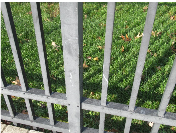
Finish deterioration
