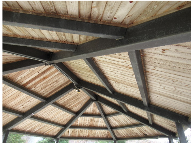
Metal roof underside
