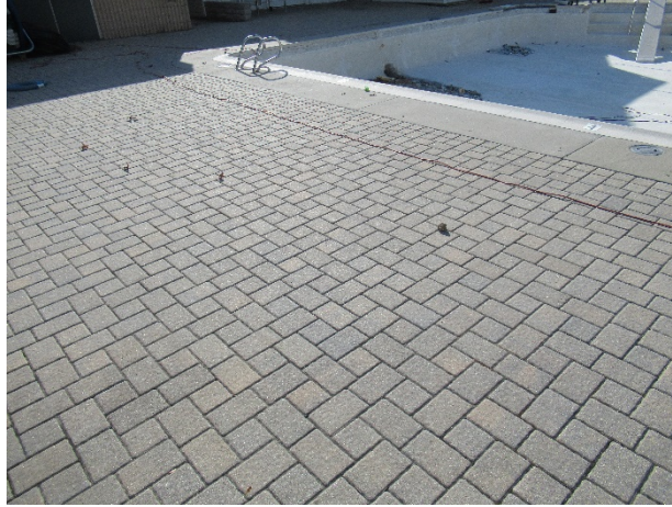
Paver pool deck overview
