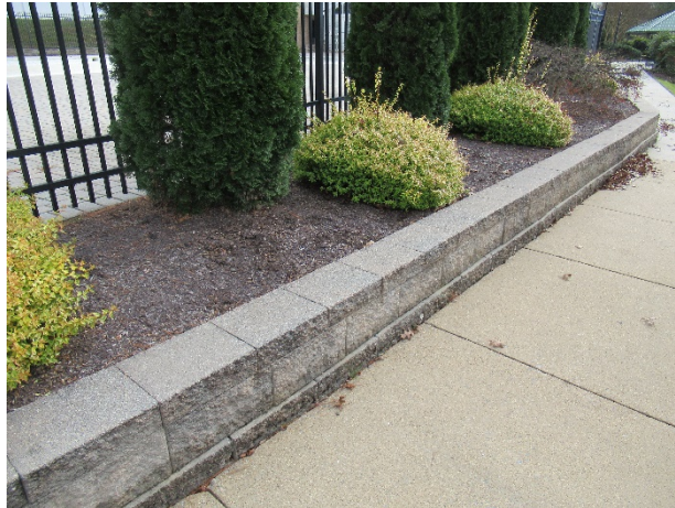
Landscape retaining walls
