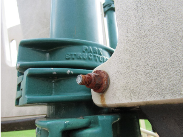
Rust at clubhouse playground
