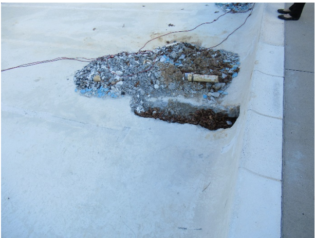
Pool overview – Note: drain removal
