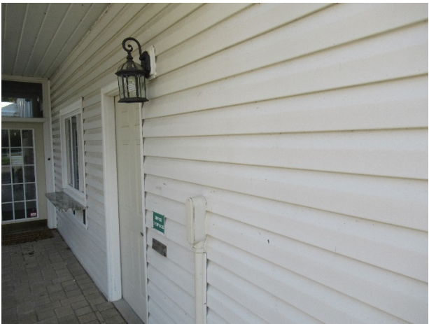
Vinyl siding overview
