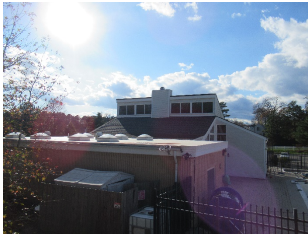
Clubhouse rear elevation overview
