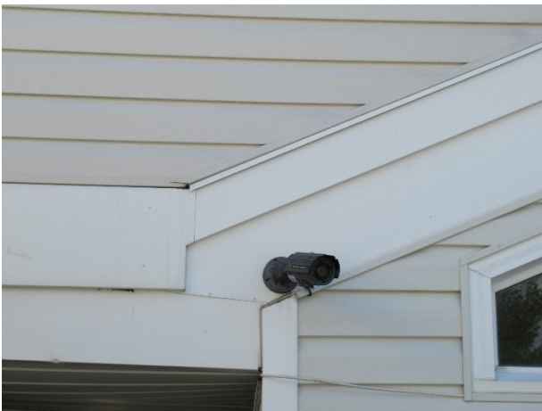
Security camera overview
