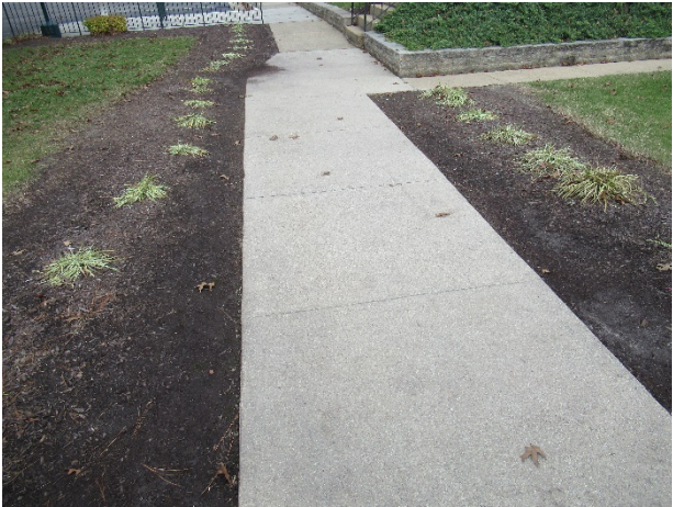
Concrete sidewalk overview
