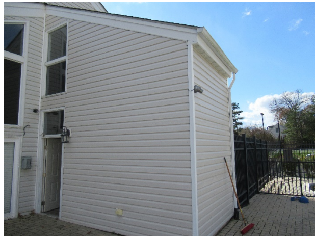
Vinyl siding overview
