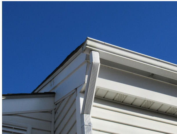
Gutter and downspout overview
