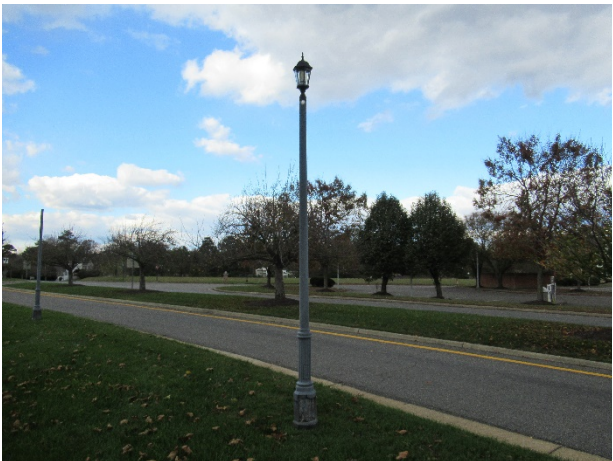
Entrance light pole and fixture overview
