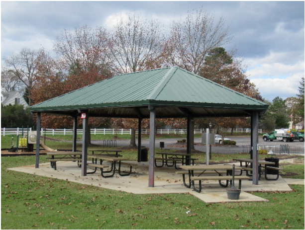
Metal roof overview
